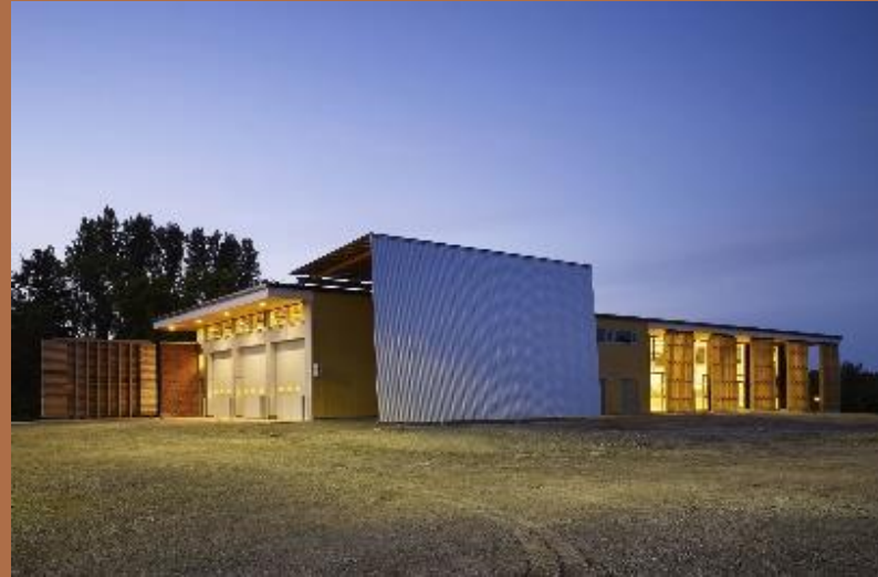
TRCA Restoration Services Building Vaughan, Ontario
